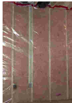
Fiberglass Insulation
